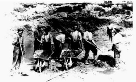
Digging down to the buried alluvial tin layer on Red Moor, Lanlivery in Cornwall c.1910 prior to using water (tin streaming) to separate the waste from the ore. Apart from the wheelbarrows little may have changed since prehistoric times (Penhallurick 1986).
