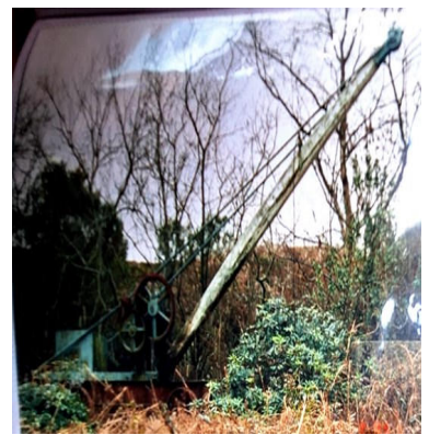
And this is an old photo of the real crane in Carbeans Quarry – thanks to J & M Grigsby
